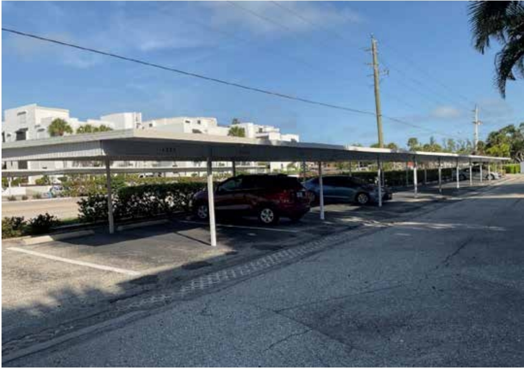
Carport, 21 Car - Bayside
