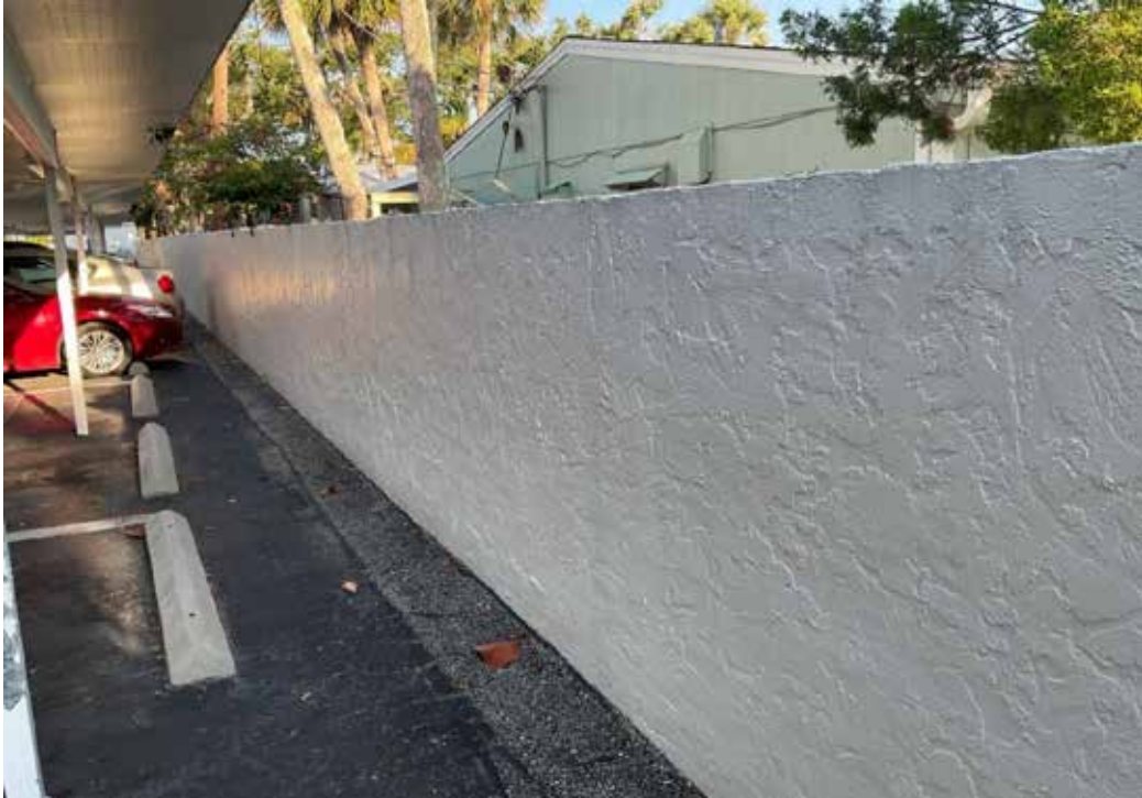
Site Wall - Bayside
