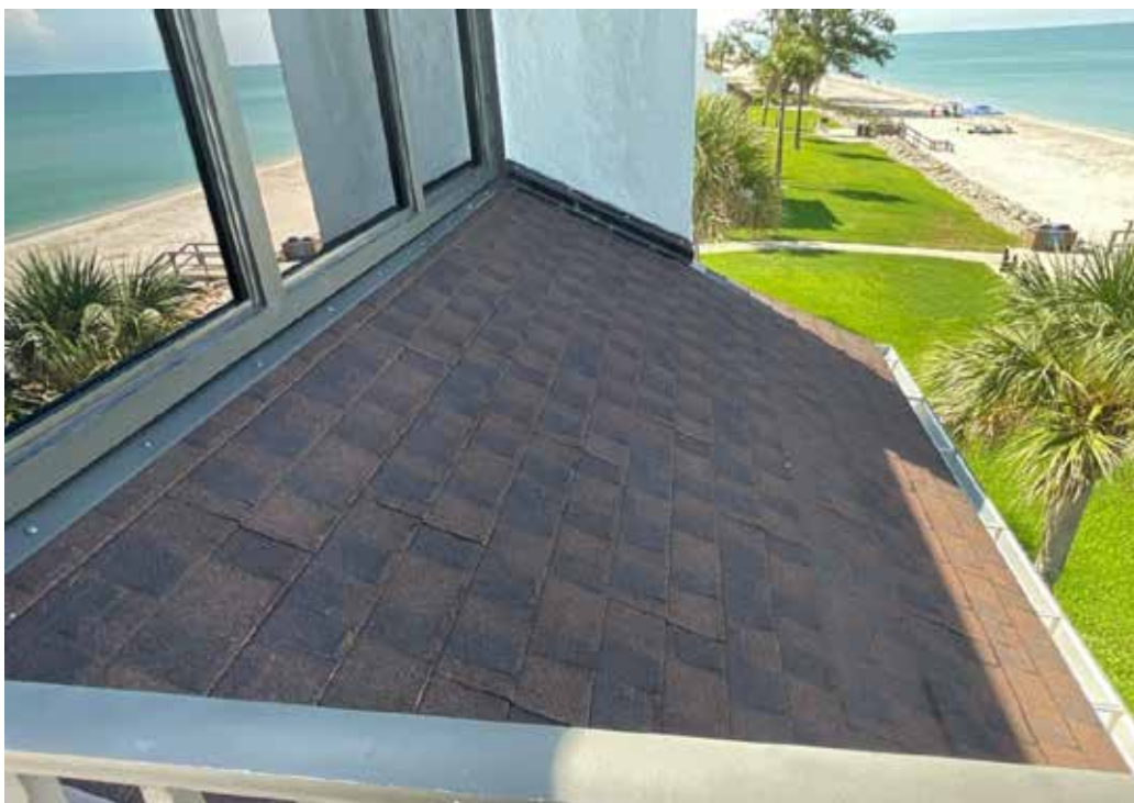
Condo Building B3 Mansard Roof
