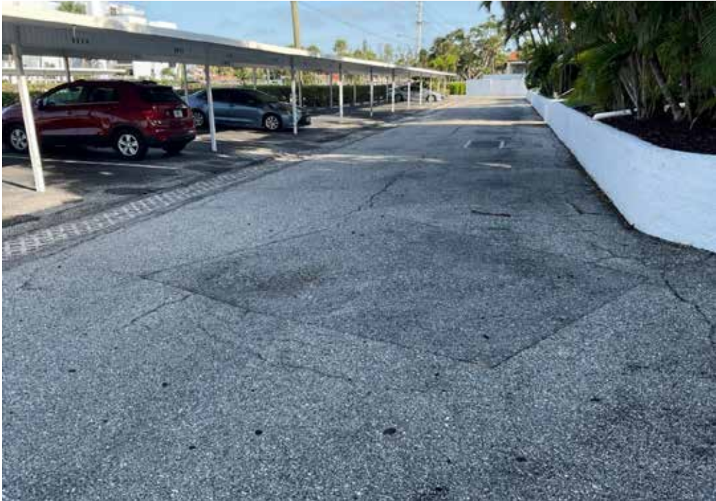
Paving, Asphalt - Bayside
