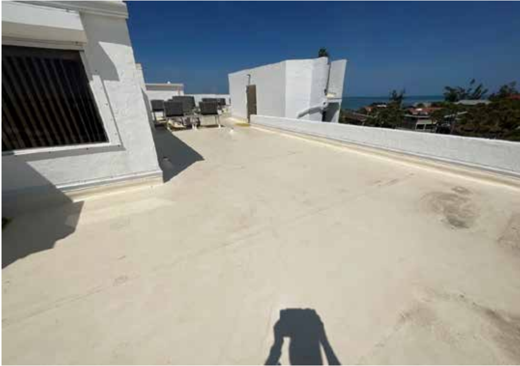
Condo Building A1 Roof
