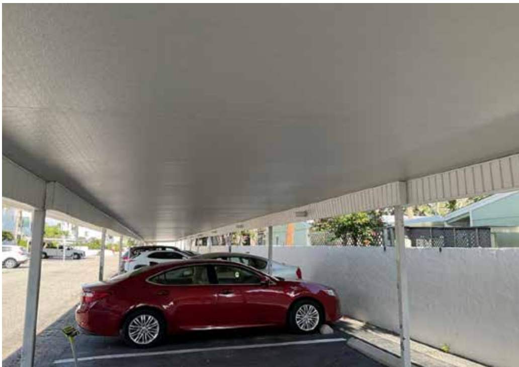
Carport Roof Panels - Typical
