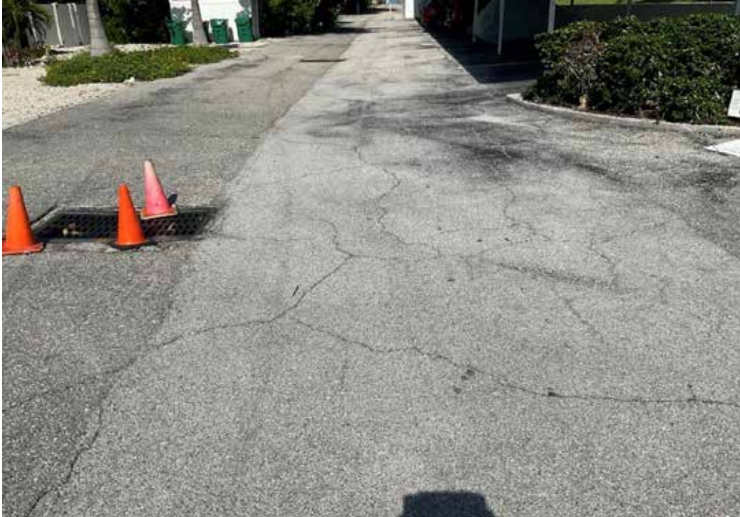
Paving, Asphalt - Gulfside
