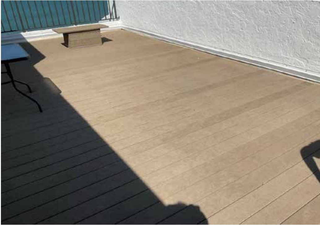
Condo Building B3 Roof Deck
