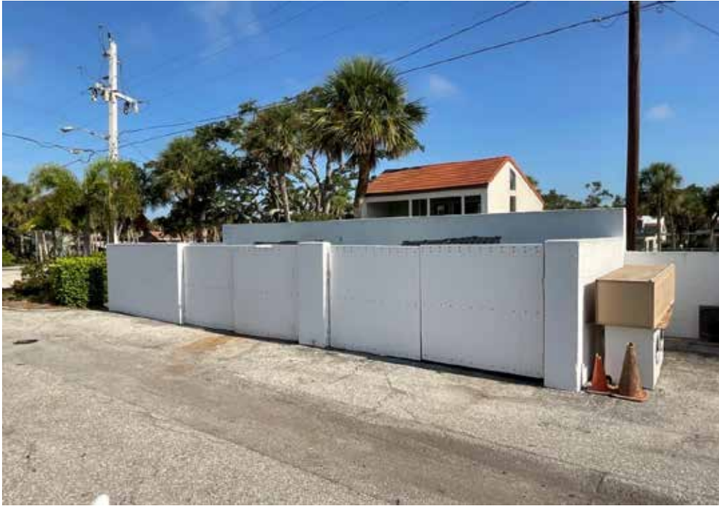
Trash Enclosure - Bayside
