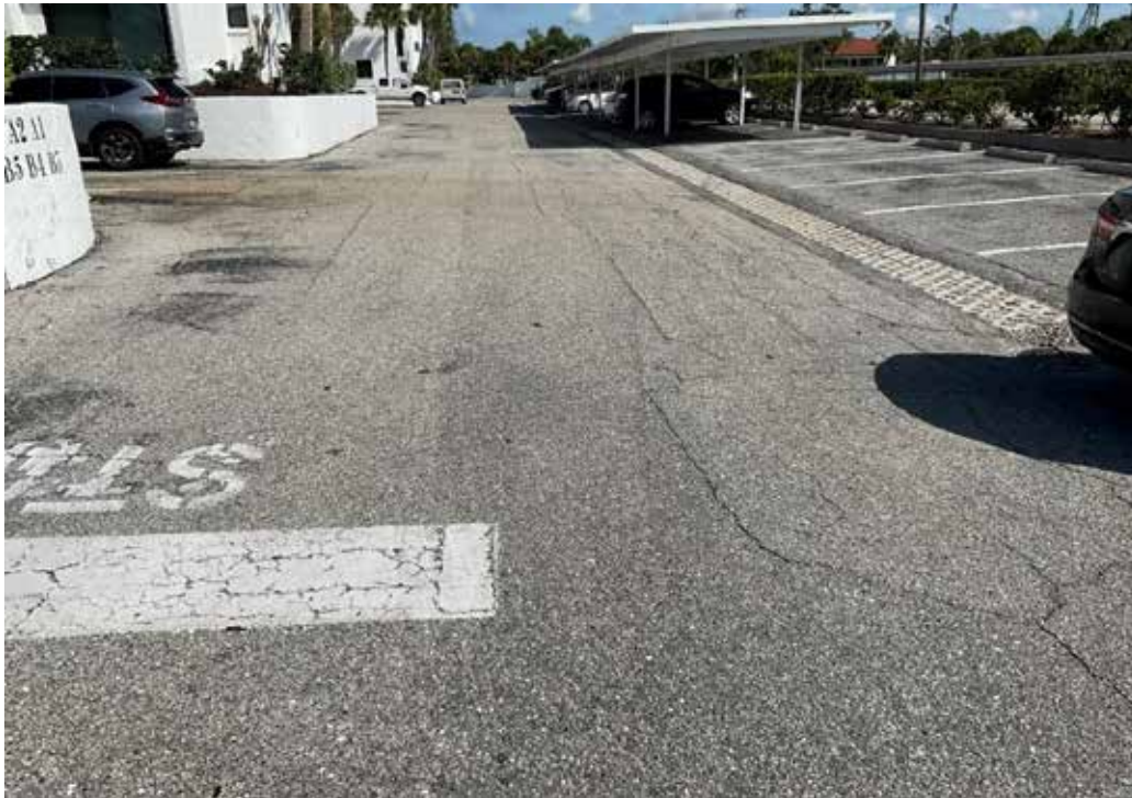
Paving, Asphalt - Gulfside
