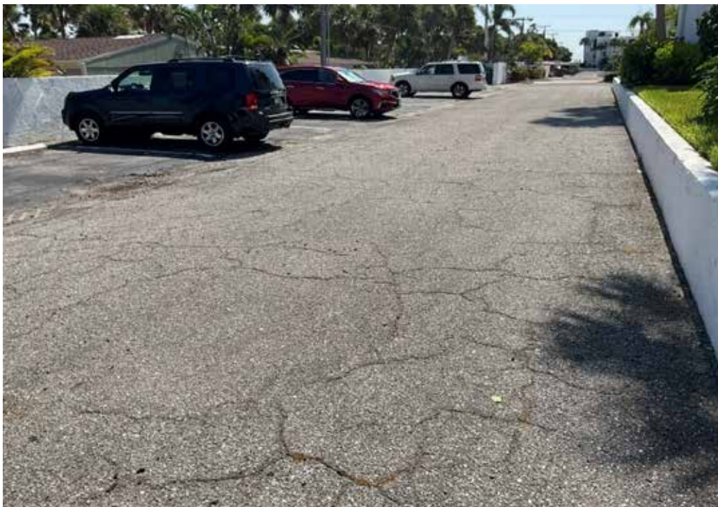
Paving, Asphalt - Gulfside
