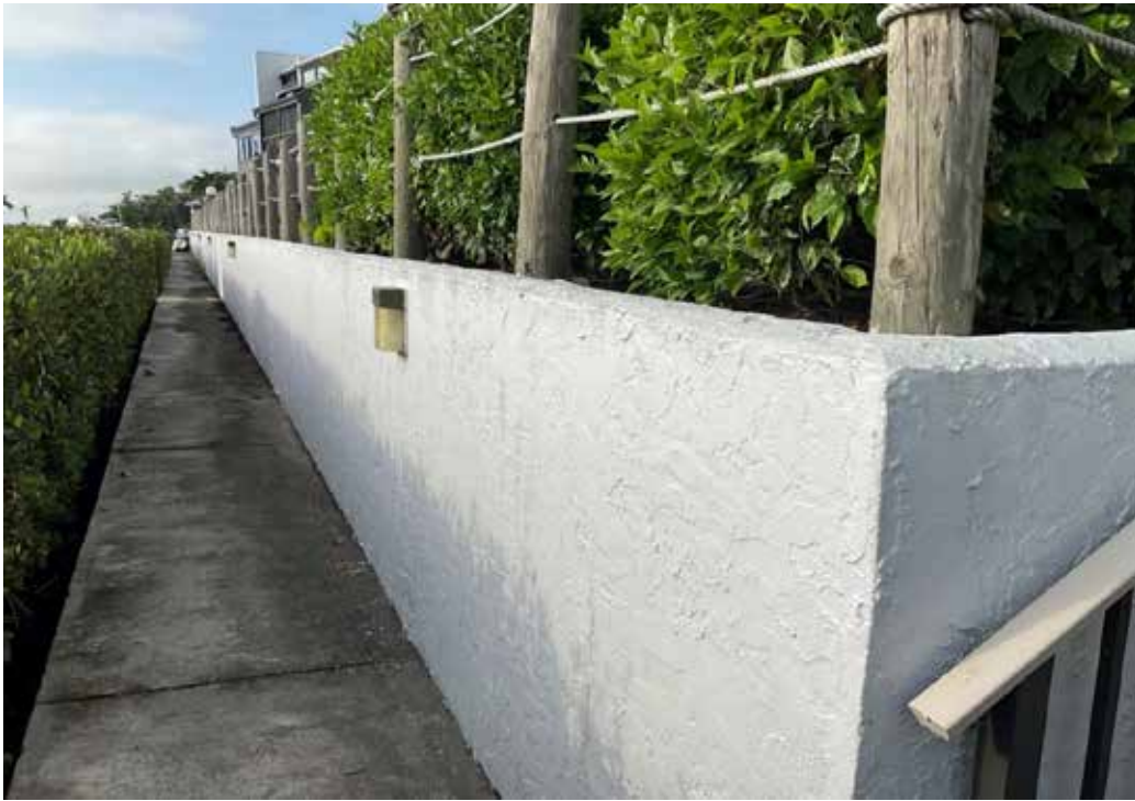
Retaining Wall - Bayside
