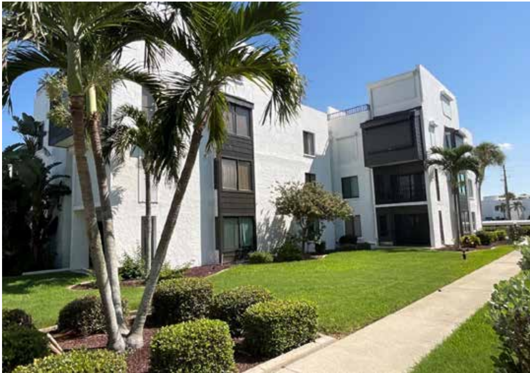
Condo Building A2
