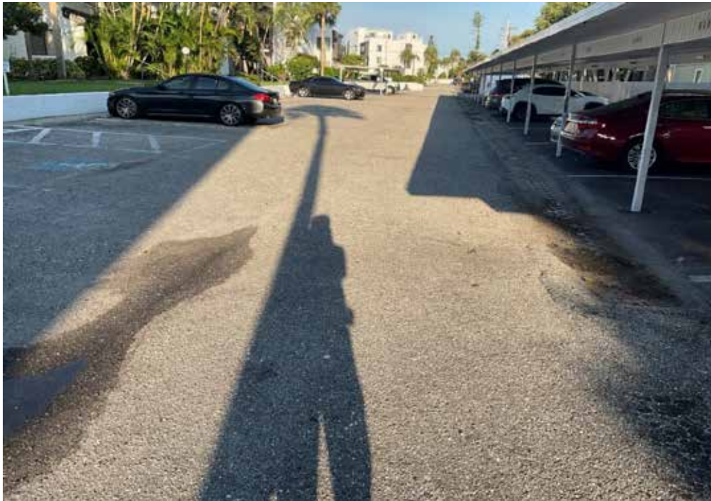
Paving, Asphalt - Bayside
