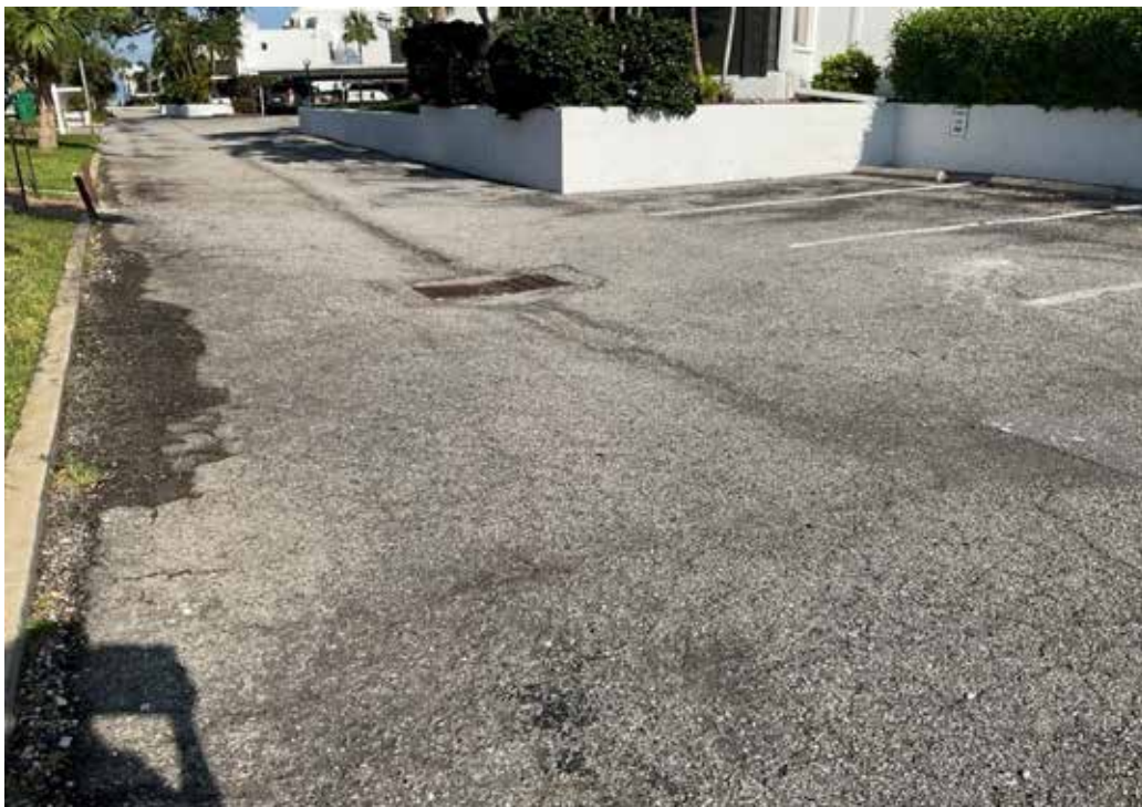
Paving, Asphalt - Bayside
