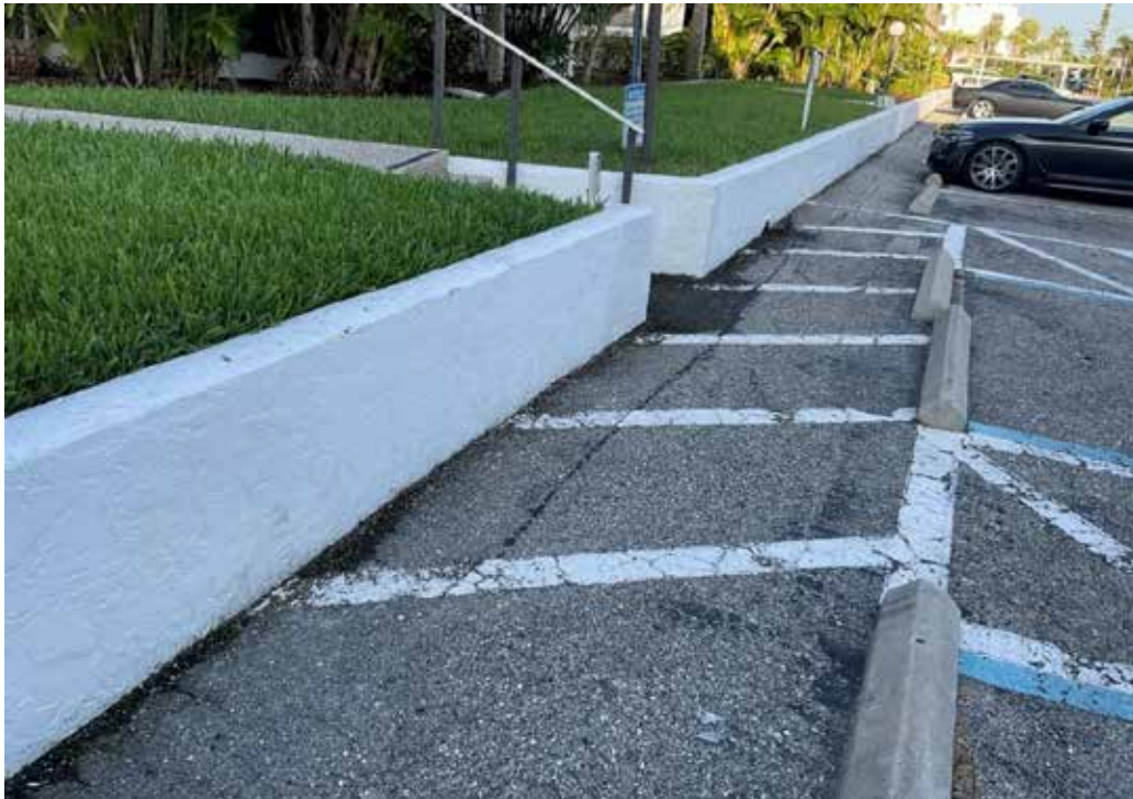
Retaining Wall - Bayside
