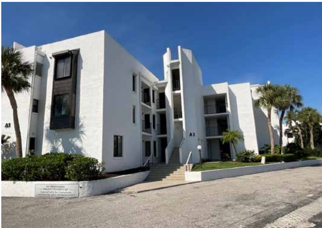
Condo Building A1
