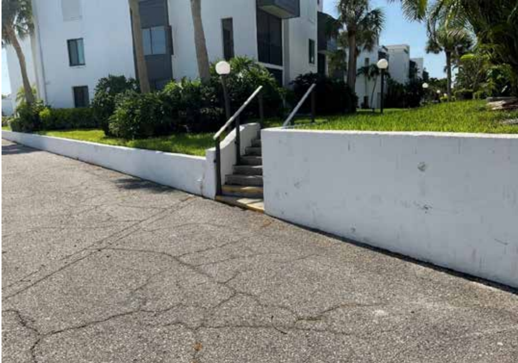
Retaining Wall - Gulfside
