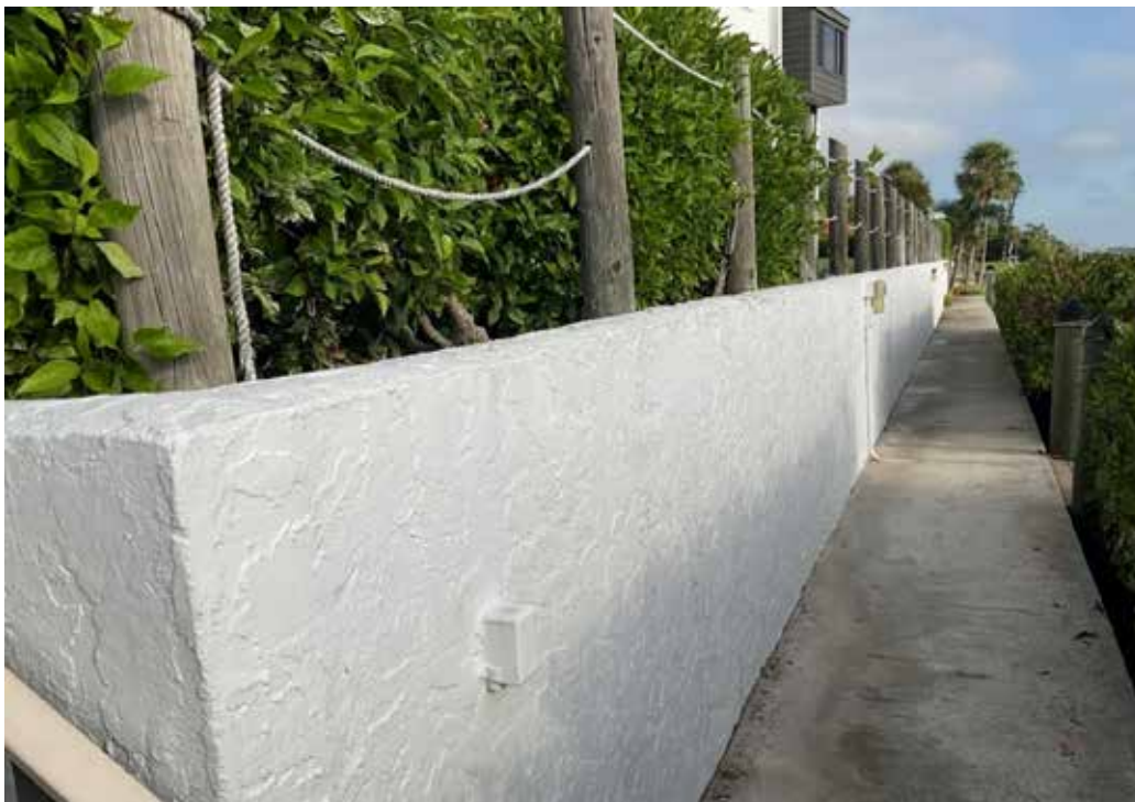
Retaining Wall - Bayside
