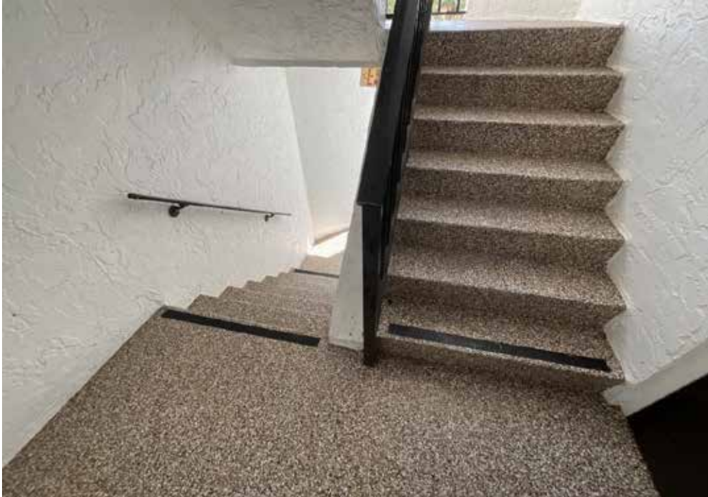
Condo Building A1 Stairwell
