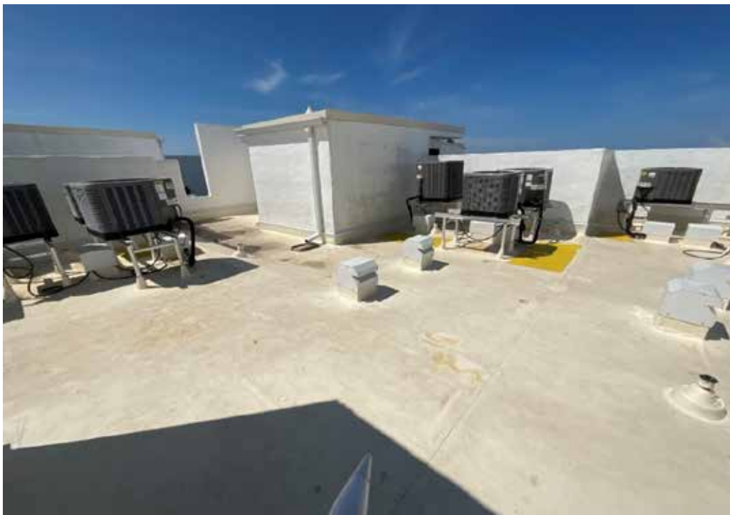
Condo Building A1 Roof
