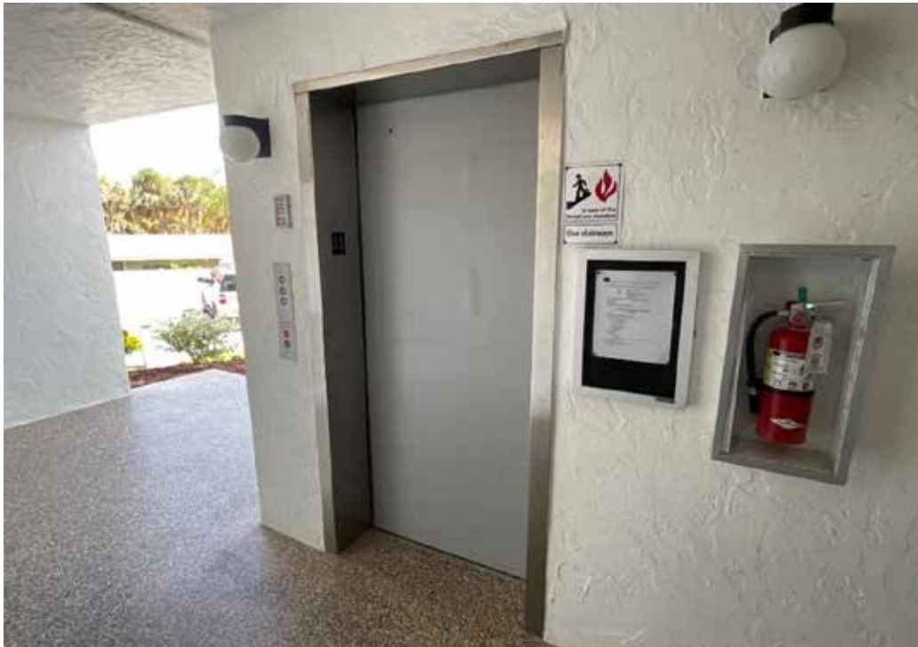
Condo Building A1 Elevator Door and Frame
