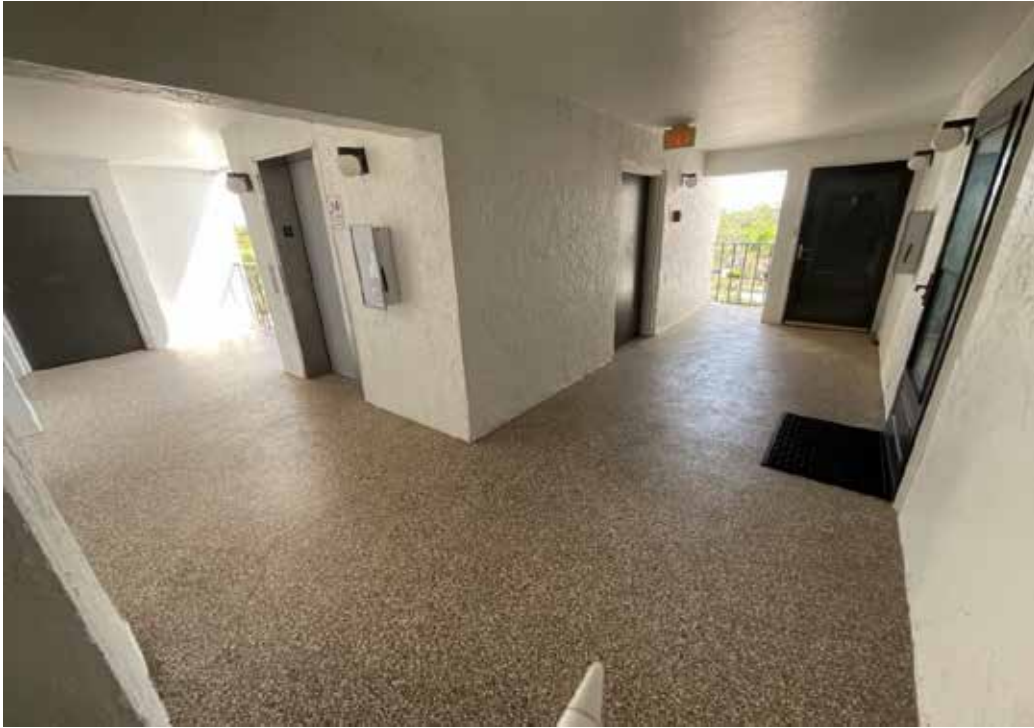
Condo Building A1 3rd Floor Walkway
