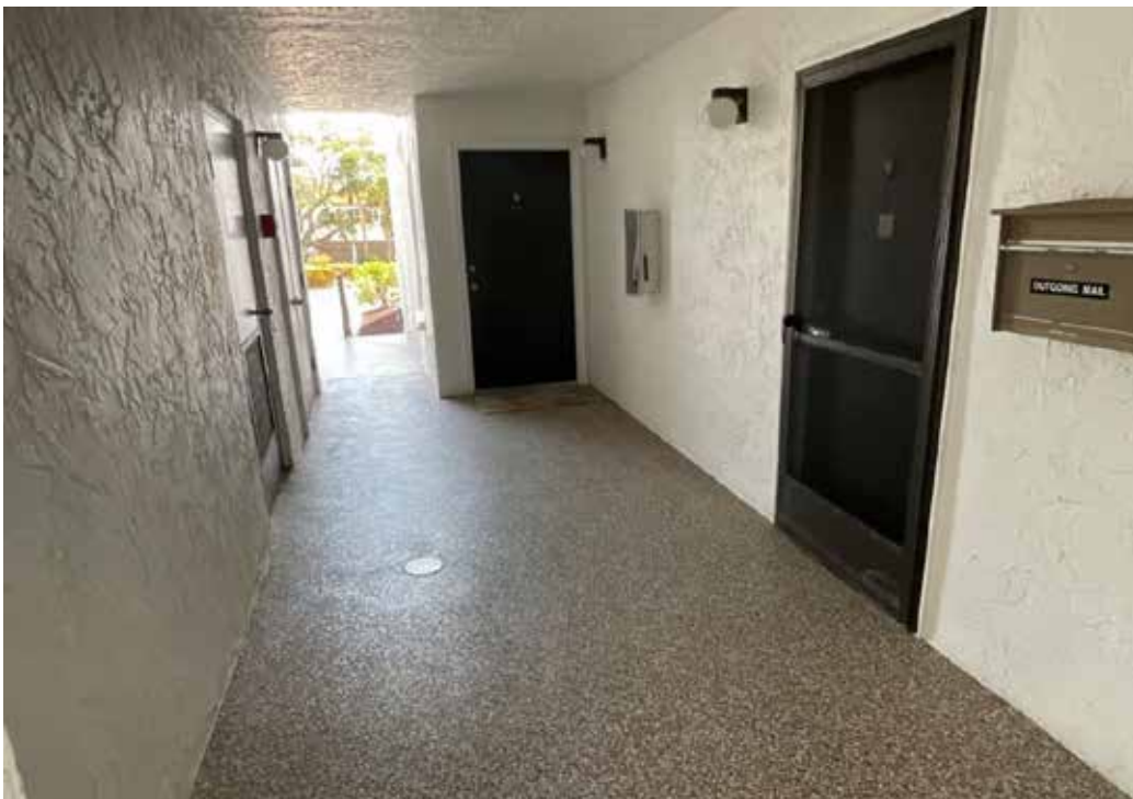
Condo Building A1 1st Floor Walkway
