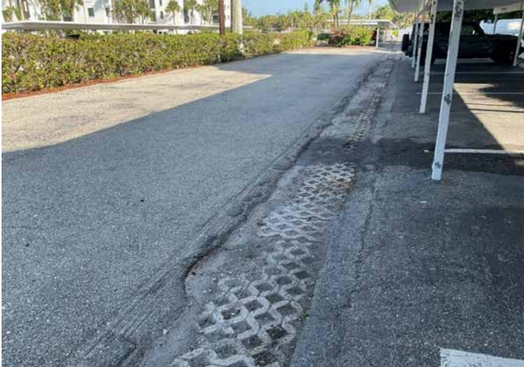
Paving, Asphalt - Bayside
