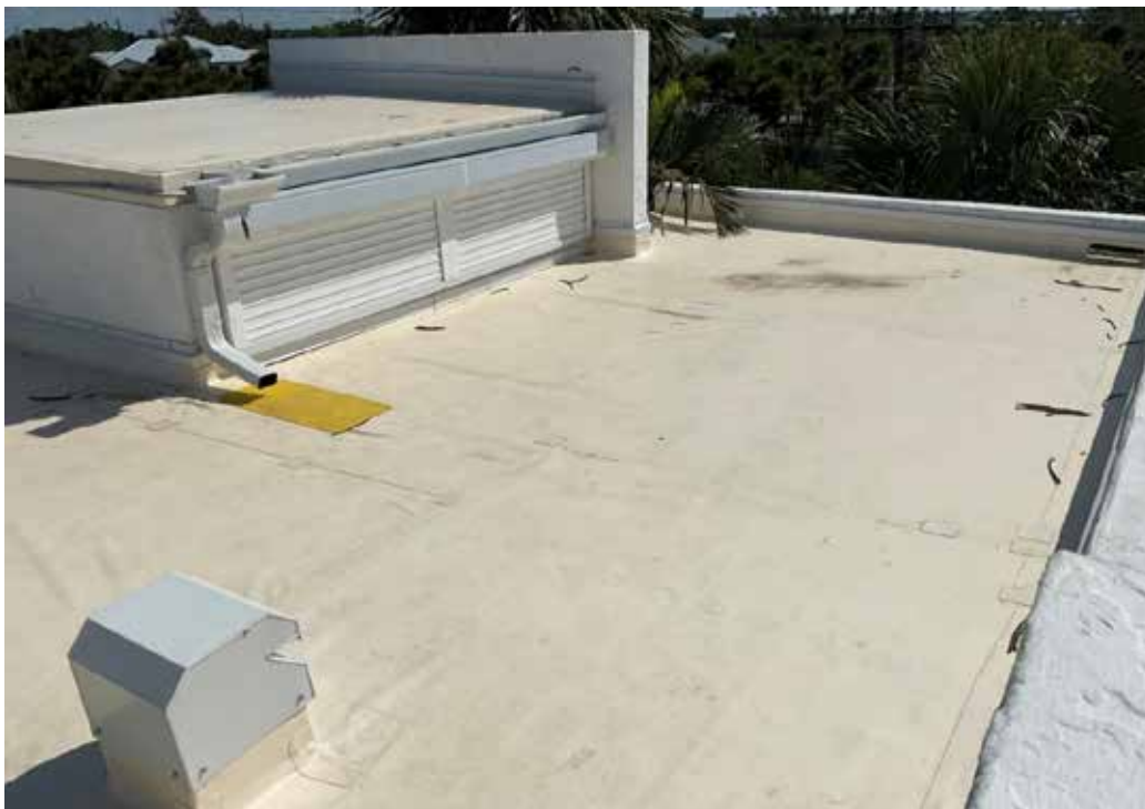
Condo Building B3 Roof
