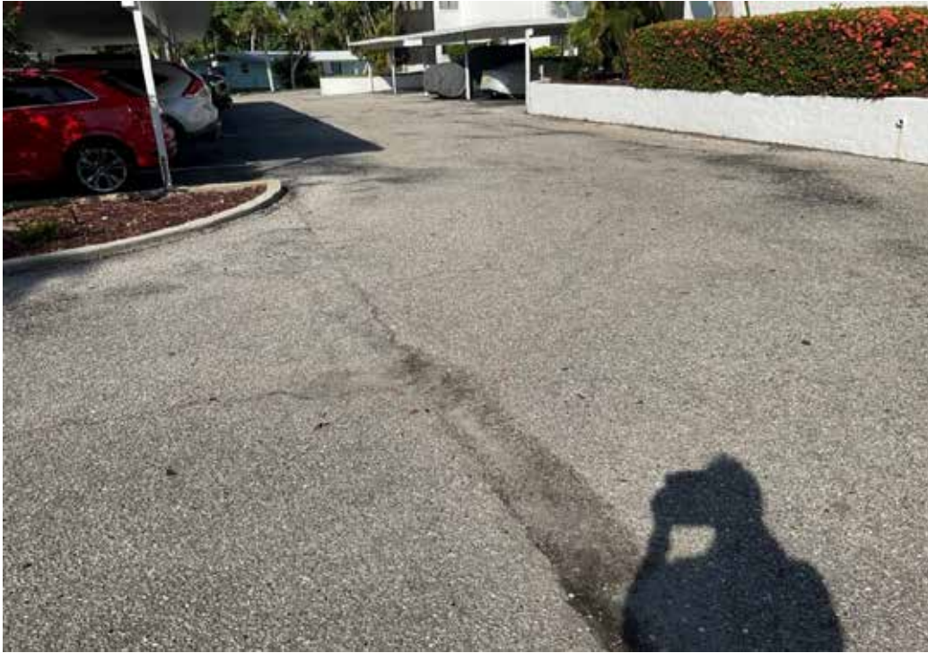
Paving, Asphalt - Bayside
