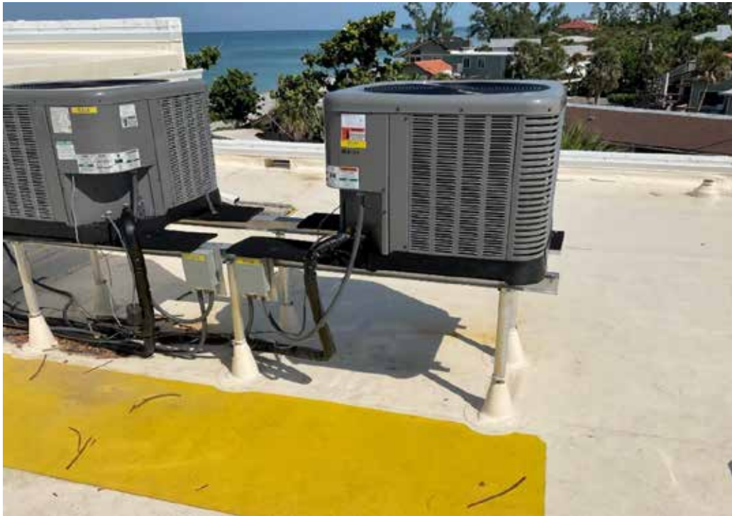
Condo Building B3 Roof
